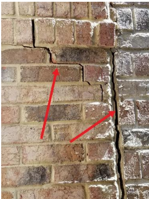
Brick step foundation has settled
