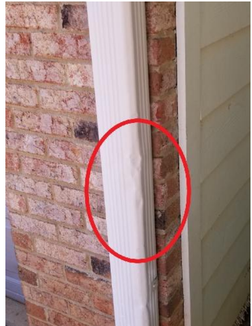
Slight damage to gutter near garage door
