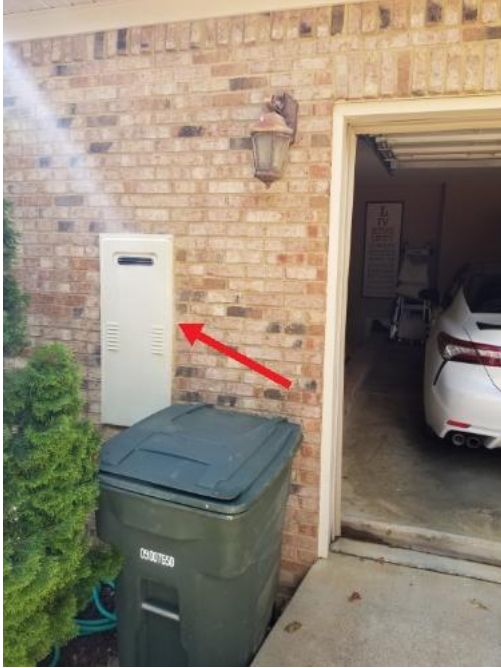
Tankless hot water heater
