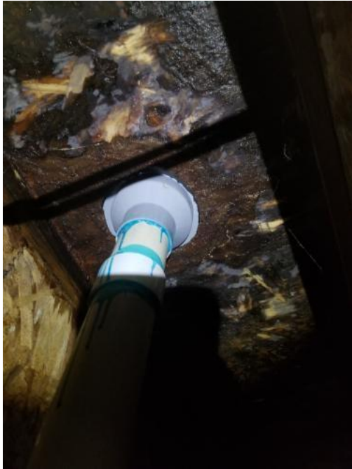
Subfloor below steam shower is leaking
