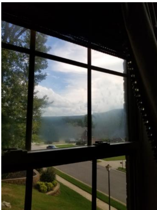
Cloudy window. Top sash has broken thermal pain
