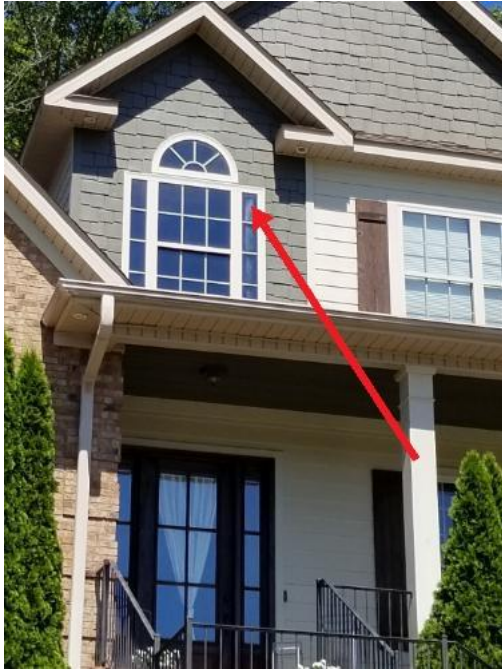
Thermal seal broken
