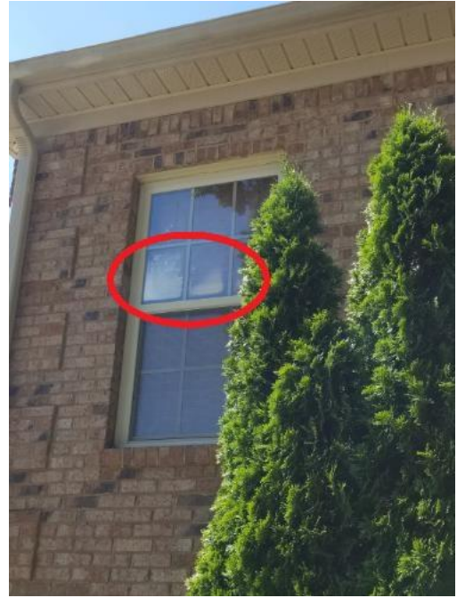
Thermal seal broken
