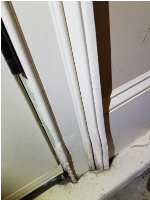
Man door casing shows some signs of water damage
