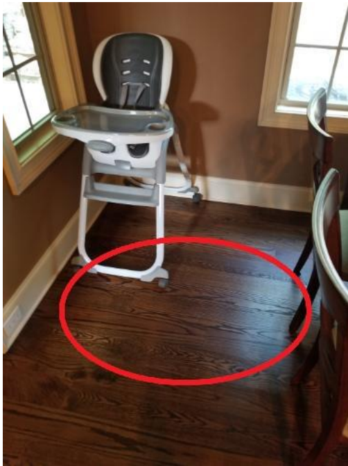
Slight warping in the floor
