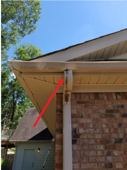
Clogged and evidence of past leaks
