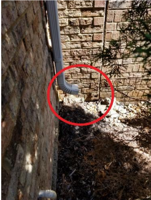
Extend gutter 4-6 feet away from house
